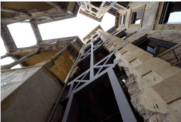
Beit Beirut or, “The House of Beirut”. The building from 1924 was partly ruined during the Civil War. It is now preserved as a museum in an attempt to include the war as part of the city's long memory. Copyright by Author.
